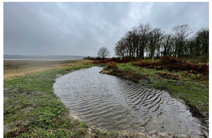
FIGURE 5 A newly constructed sediment pond at Warren Mill. Credits: LIFE WADER.
