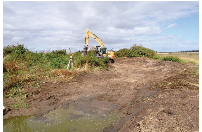
FIGURE 4 Construction works at the sediment ponds at Warren Mill. Credits: LIFE WADER.
